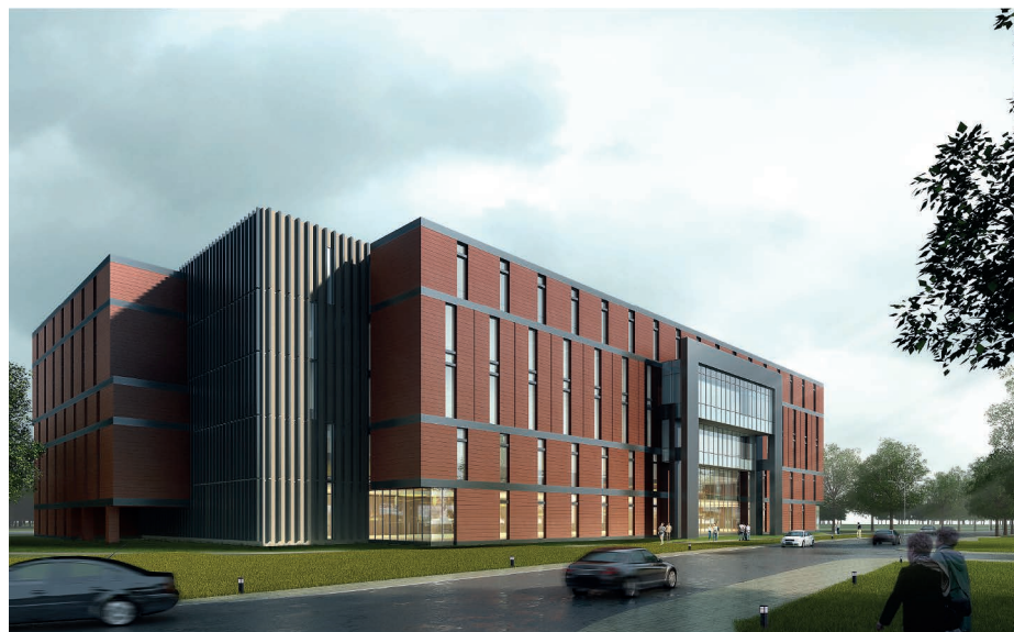
Figure 1 | An artist's impression of the Center for High Pressure Science and Technology Advanced Research headquarters that is currently under construction in Beijing (due to be completed in October 2017).
